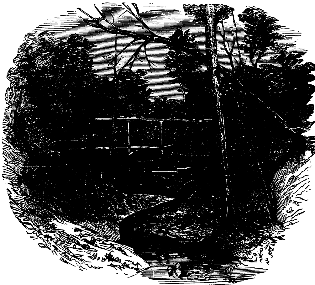
HIGH BRIDGE, LAKE BLUFF, LAKE COUNTY, ILLINOIS.
